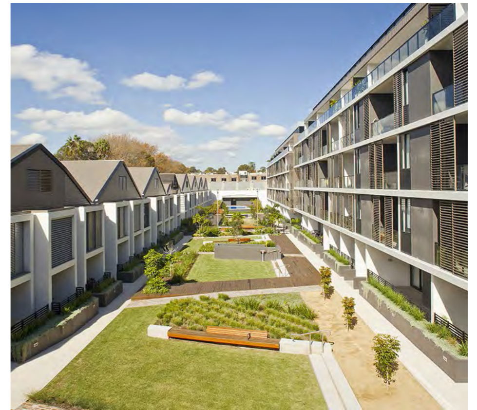
Gantry Apartments, Sydney
