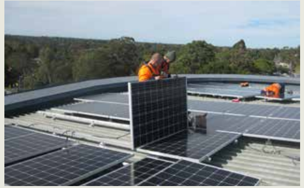
Solar PV panels being installed
