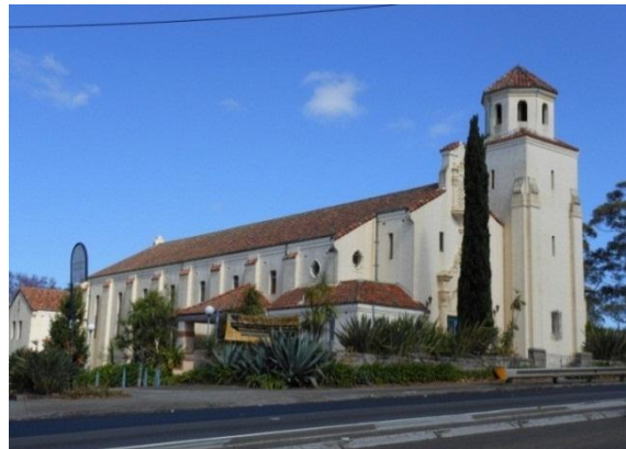
Figure 5: ‘Ku-ring-gai Town Hall’, (former Sacred Heart Catholic Church site), at No 1186 Pacific Highway, Pymble, is significant as a local landmark and as a good example of Inter-war period (c1934), Spanish Revival style of architecture.
