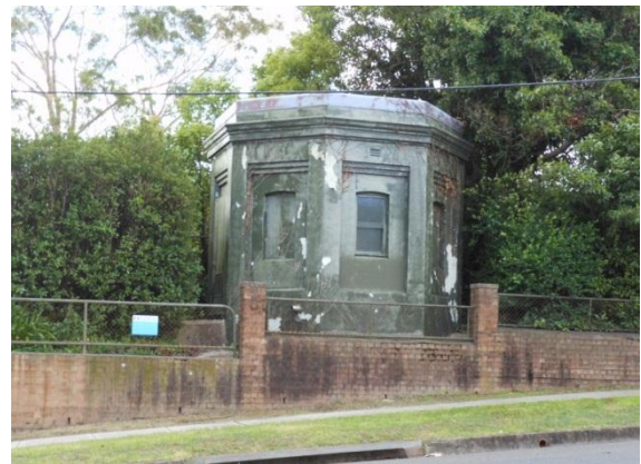
Figure 11: ‘Pymble Reservoir’ (Covered), at No 2C Telegraph Road), Pymble, built wholly of concrete in c1900, is significant demonstrating the broad range of construction techniques and the high level of technical expertise available to the Metropolitan Water Sewerage and Drainage Board (MWS&DB), to meet the demands of the increasing population of the North Shore in the early 20 th century. The site comprises a fine valve house and retains the original valve control gear.
