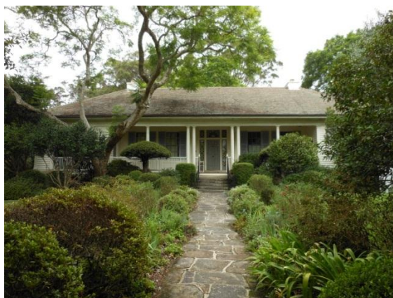
Figure 10: 'Erydene', at No 17 McIntosh Street, Gordon, built in 1913, is significant for its collection of Camellias, gathered by Professor Eben Gowrie Waterhouse (1881-1977). Waterhouse founded the Australian Camellia Research Society in 1954 and the International Camellia Society in 1962. The collection remains a resource for the future study of the genus.
