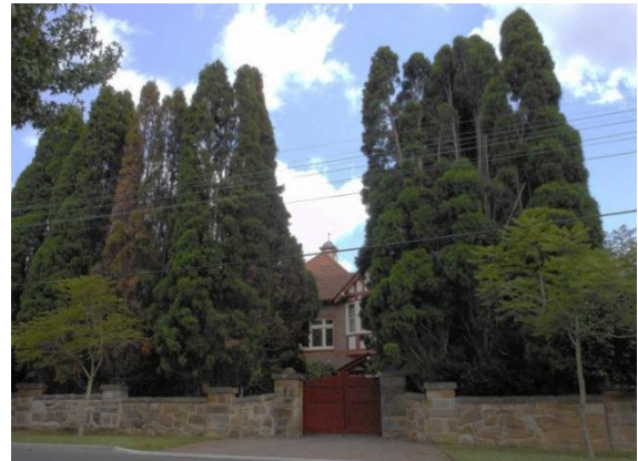
Figure 3: ‘Ingleholme’, at No 17 Boomerang Street, Turramurra, built in c1895, is significant for its association with prominent Architect and Town Planner Sir John Sulman (1849-1934). Sulman lived at the house for some 16 years and undertook several extensions.
