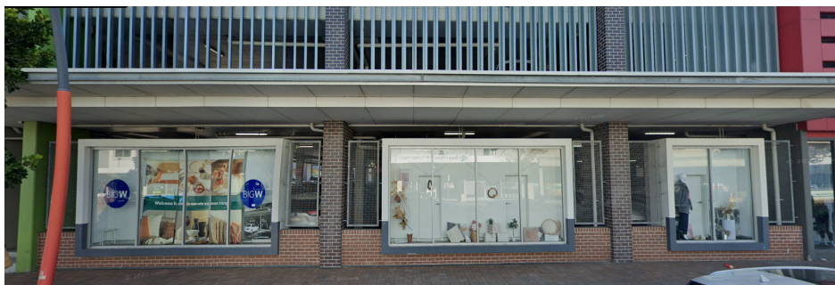
Figure 14G.5-2: Example of above ground car parking sleeved with glazed display cases
