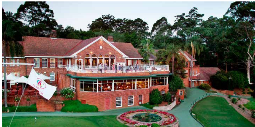
Figure 14I.1-2 Photo of Heritage Item Clubhouse
