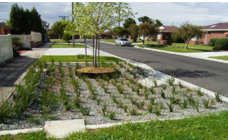
Figure 3A.5-2. Raingarden retrofit to roadway - Mentone, Melbourne (www.wsud.org)
