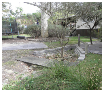
Figure 24C.6 -2 A local raingarden connected to the overflow of a rainwater tank improves water quality and reduces runoff to the adjoining bushland.
