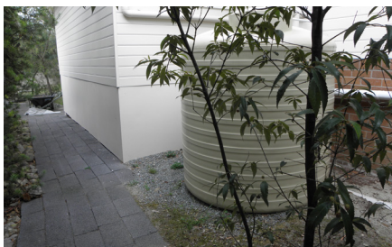
Figure 24C.4-1 Rainwater tank blends with dwelling
